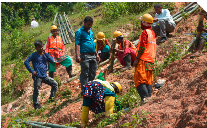
Bio-engineering work for slope stability.
