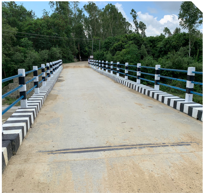
Maintained crossing structure.
