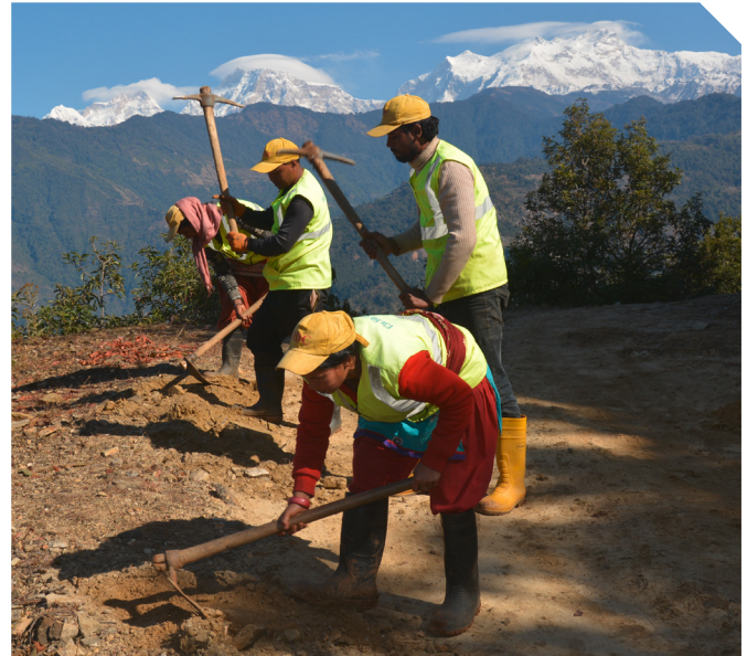
Rural road maintenance carried out by RMG members
