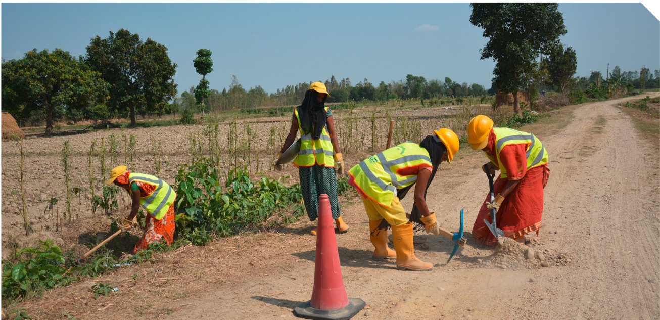
Women Road Maintenance Group at work
