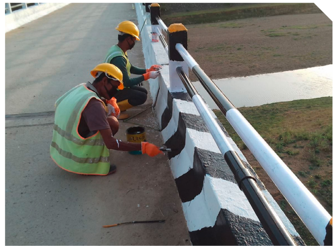
Maintenance works under SNRTP
