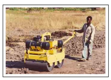
standards, acceptable levels of deviation, and schedules of penalties (e.g. deductions), when certain standards are not met. Special attention should be given to the compaction of ETL. Especially where deep ruts were filled with borrow material, care must be taken to compact in sufficient thin layers so that uneven settlement at a later stage will be avoided.
