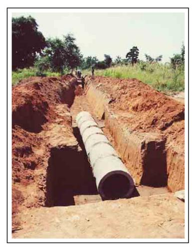
Picture 31: Culvert trench and in- and outlet excavation, at Kijuka - Nyamahona road, Sengerema District, Tanzania.
