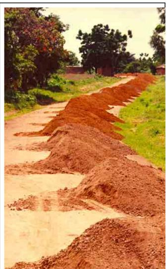
hand, as for trailers. Gravel dumps lined up on the road as shown in Picture 65, may be the correct practice for a Machine Based implemented contract, but is bad practice for a Labour Based implemented contract for following reasons:
