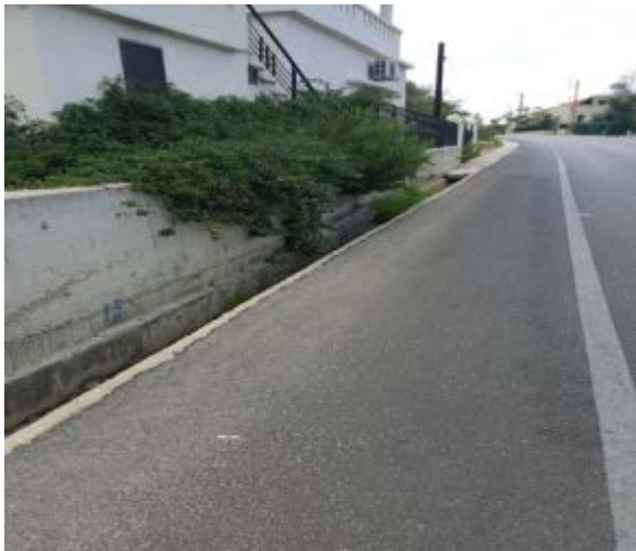
Saadiyyat Project - Road after rehabilitation
