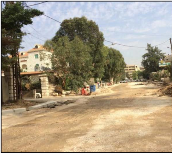
Hazmieh Project - Surface works
