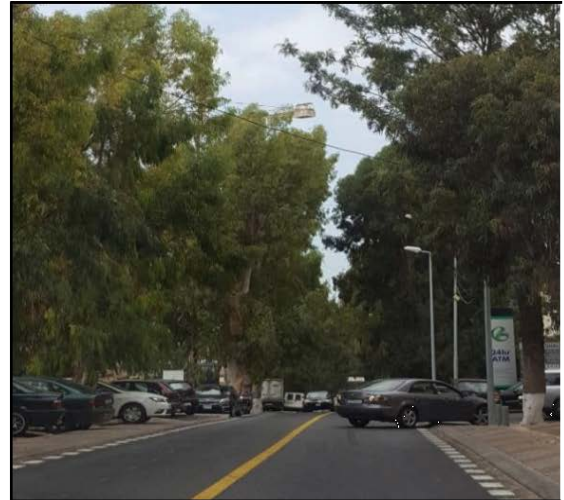
Hazmieh Project - Road after rehabilitation
