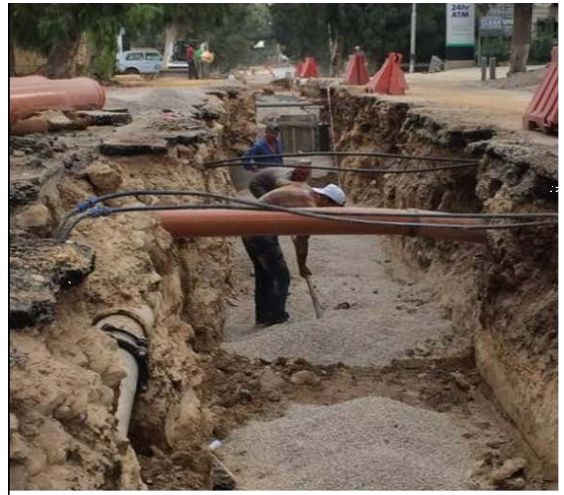
Hazmieh Project - Water and wastewater network
