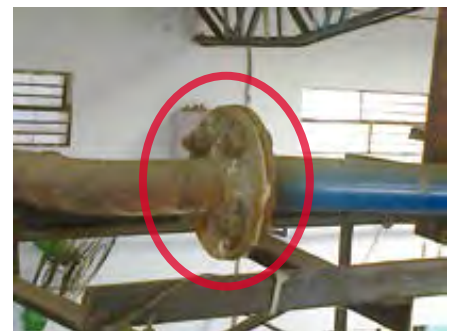
Air leakages plugged
