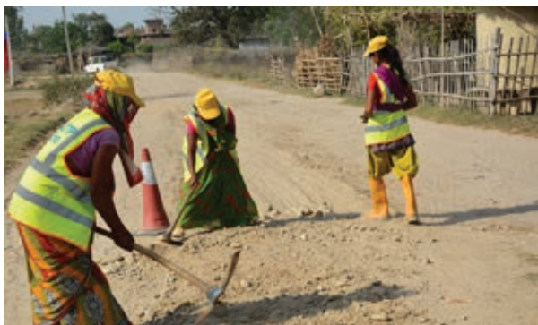
Repairing ruts and potholes
