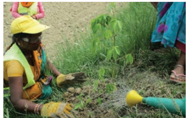
Protection of slopes by planting vegetation
