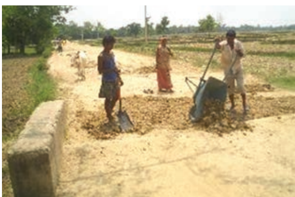
Repairing retaining walls
