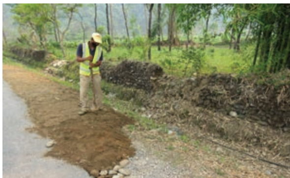
Repairing the road shoulder
