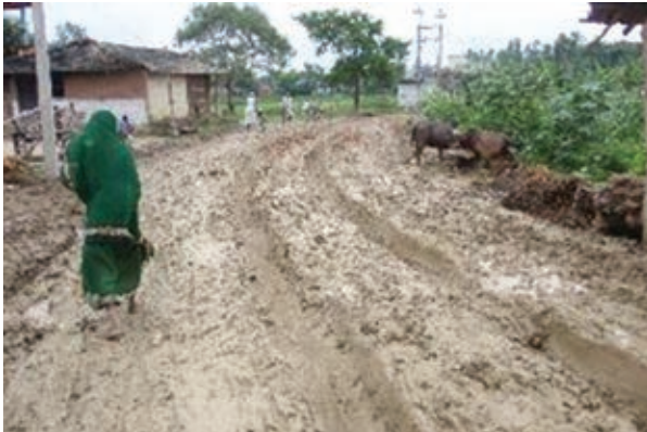
Rut formation in waterlogged areas
