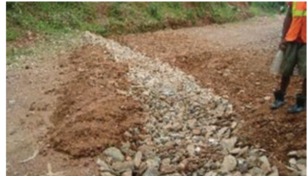
Creation of stone paved water crossings
