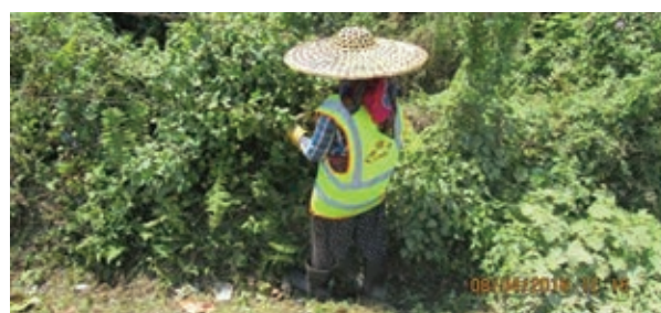
Clearing & maintaining culverts
