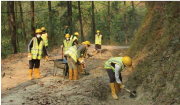
Creation of side drains
