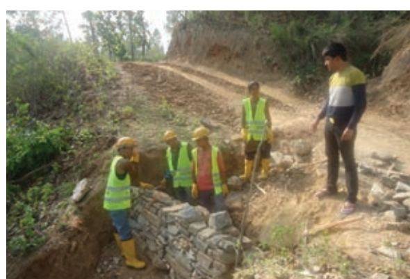
Repairing the backfill over culverts
