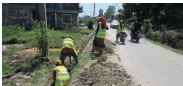
Clearing and cutting vegetation
