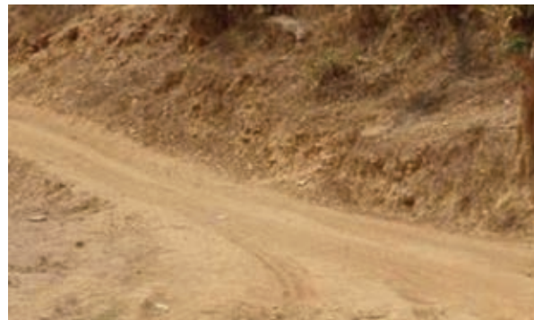
Pothole formation by vehicles
