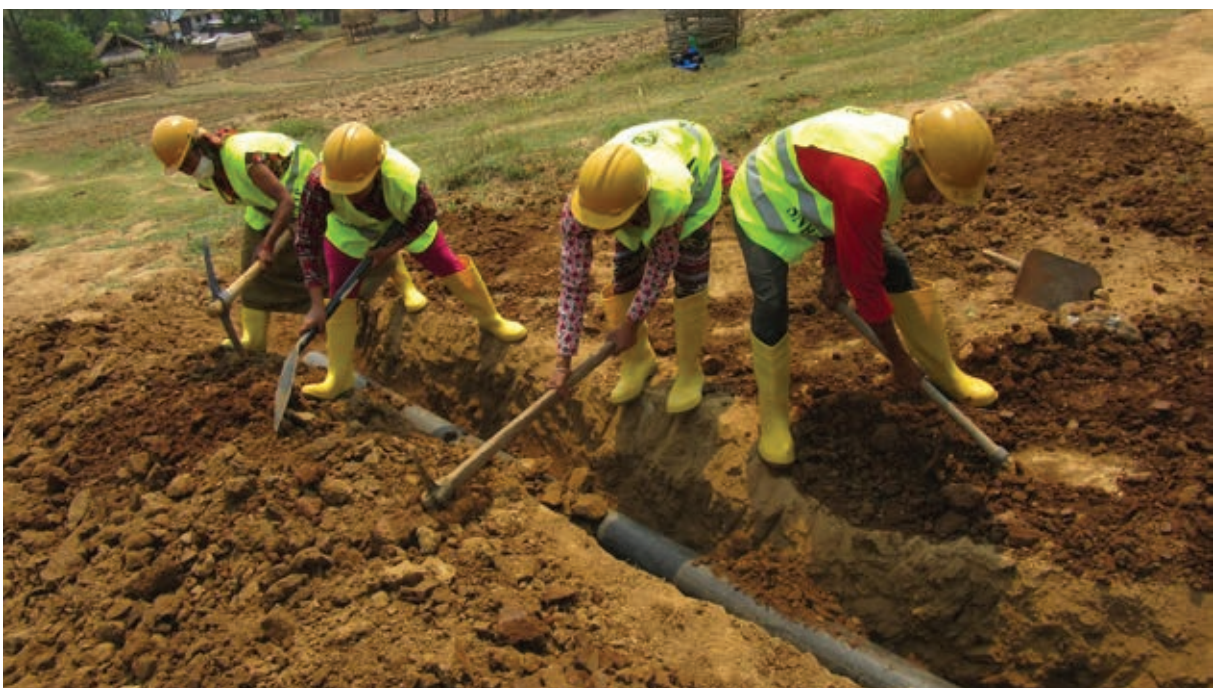
RMG members working for cross drain
