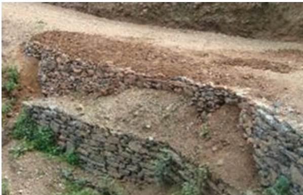
Creation of dry stone retaining walls
